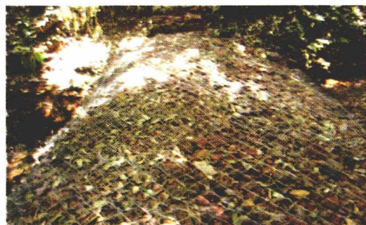
DRY STONE MESH GABION BUND FOR WATER HARVESTING
