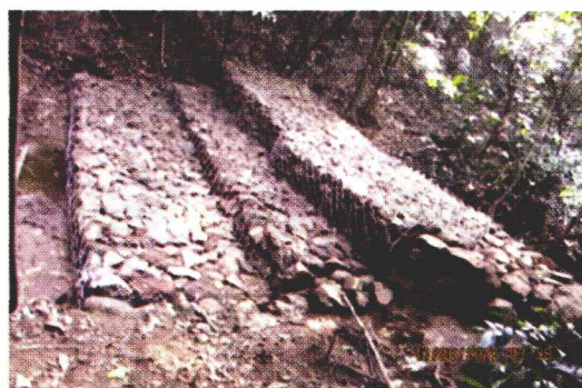
GABION CHECK DAM FOR WATER HARVESTING, SIMILIPAL TIGER RESERVE
